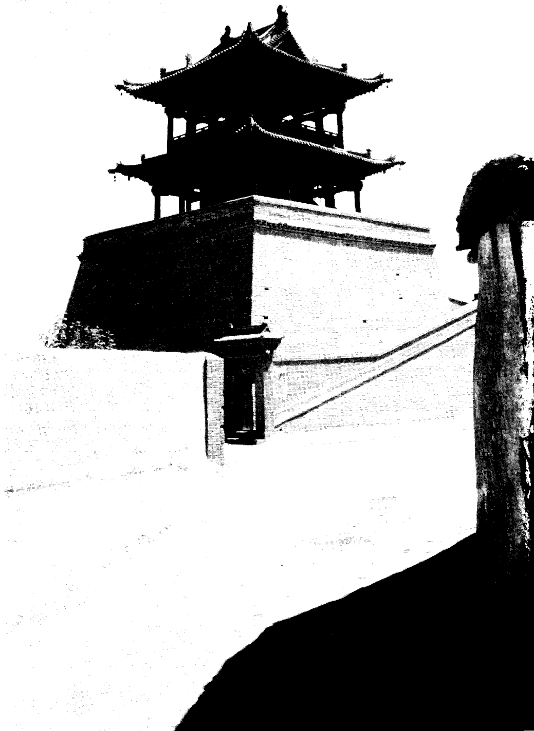
A drum tower in Wuwei, built during the T'ang dynasty, rebuilt during the Ming dynasty, and restored during the Ch'ing dynasty. It is now a provincial monument.
